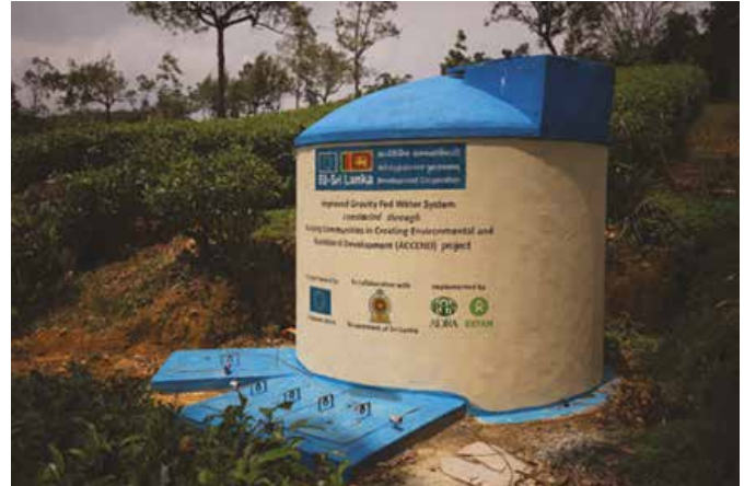
New Water Project- Fairlawn Estate
