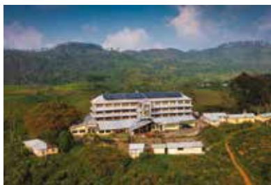
Solar Project - Gouravilla Tea Factory
