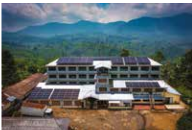
Solar Project- Stockholm Tea Factory
