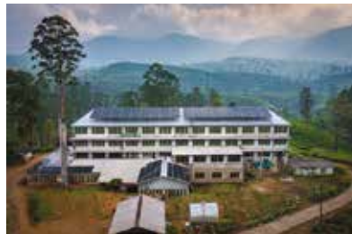
Solar Project- Mahanilu Tea Factory
