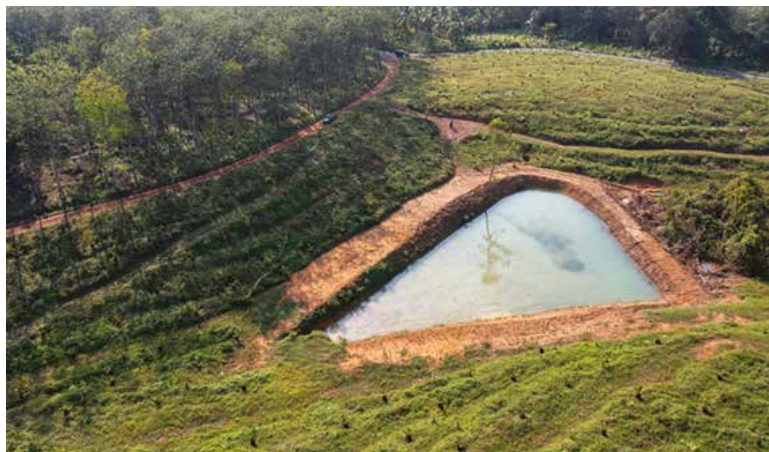
Rainwater Harvesting - Hillstream Estate
